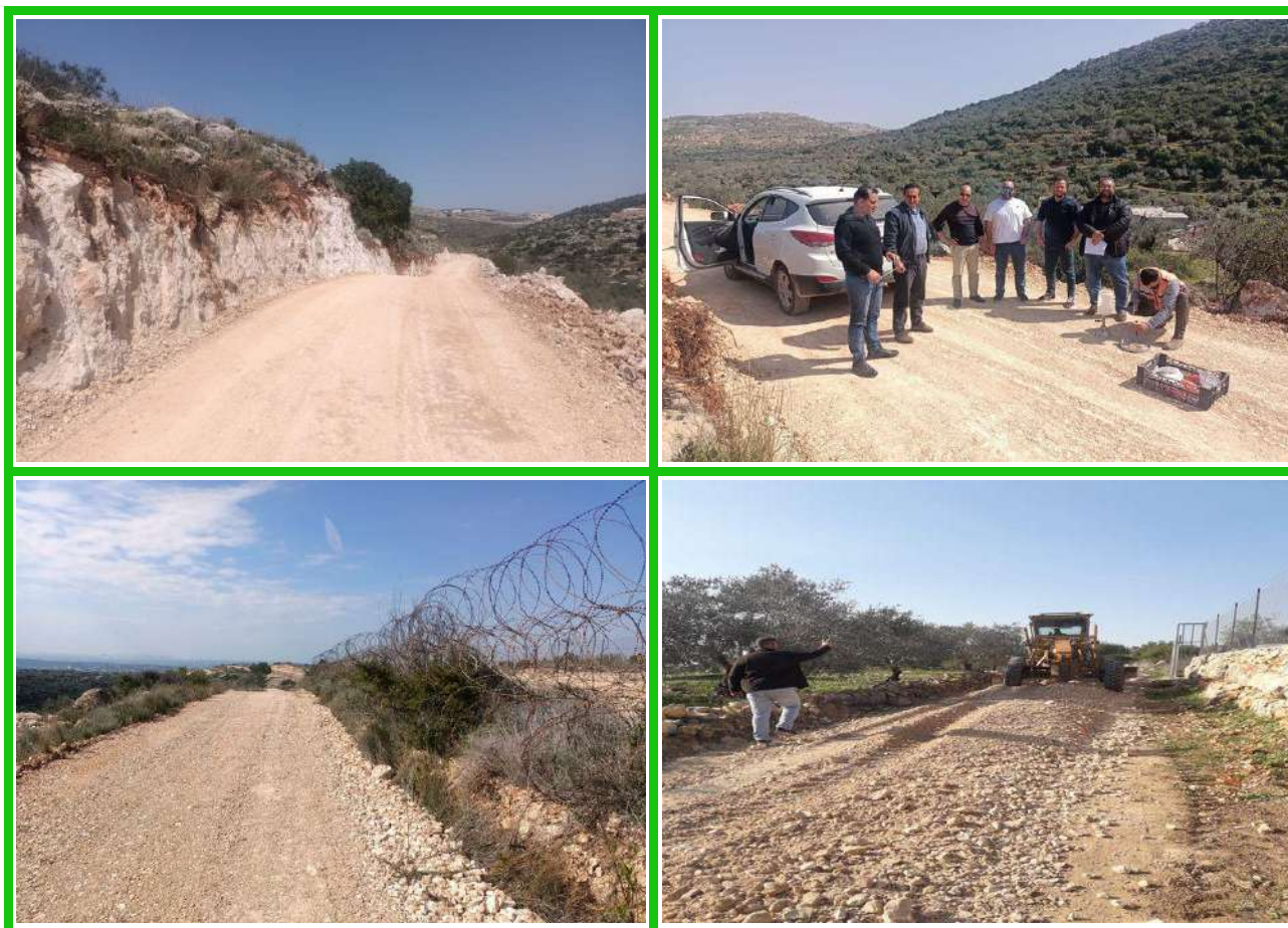
Some photos of road rehabilitation
